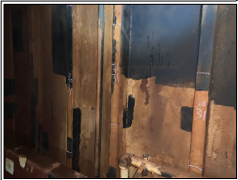
MIDDLE SECTION OF STIFFENERS PREVIOUSLY RENEWED LOOKING FORWARD
