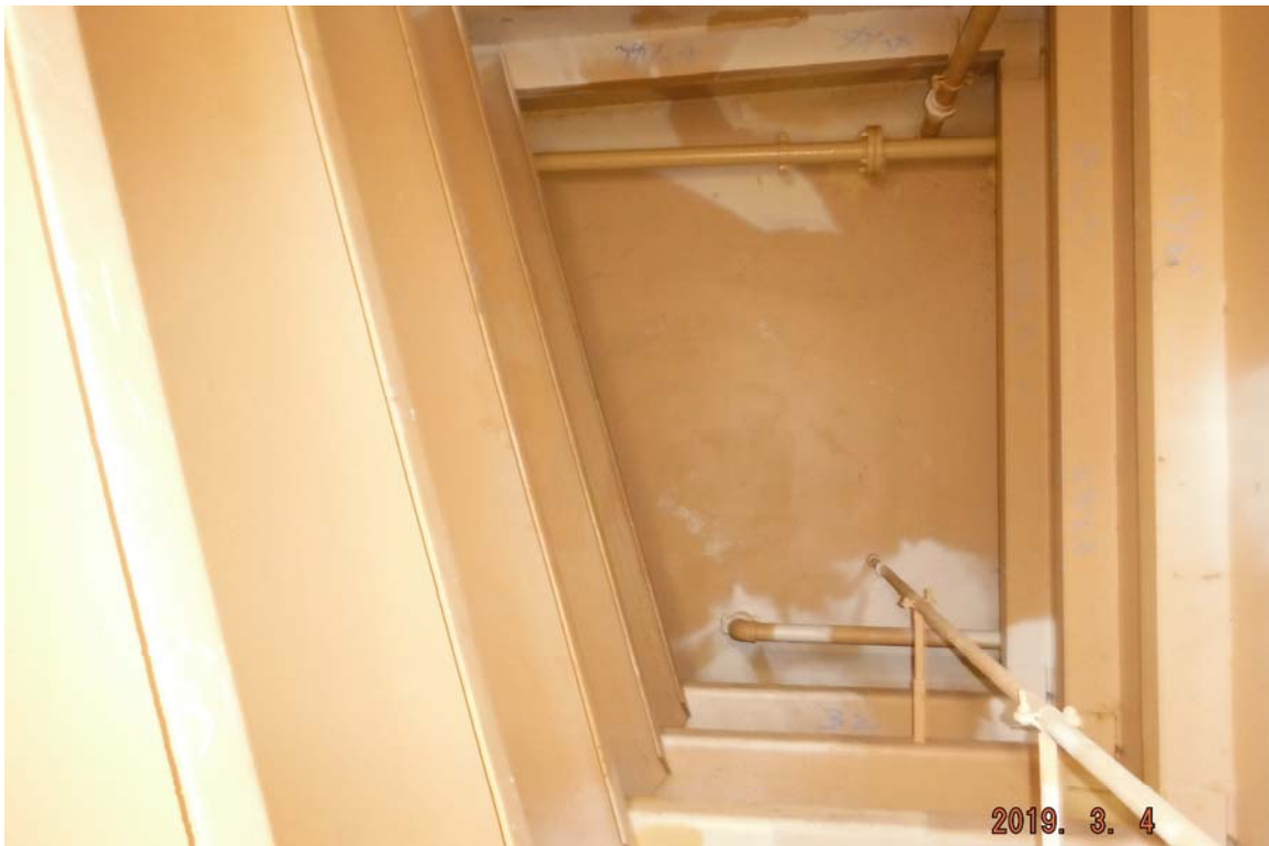
Photo No. 6 Interior void, representative sample of internal coatings
