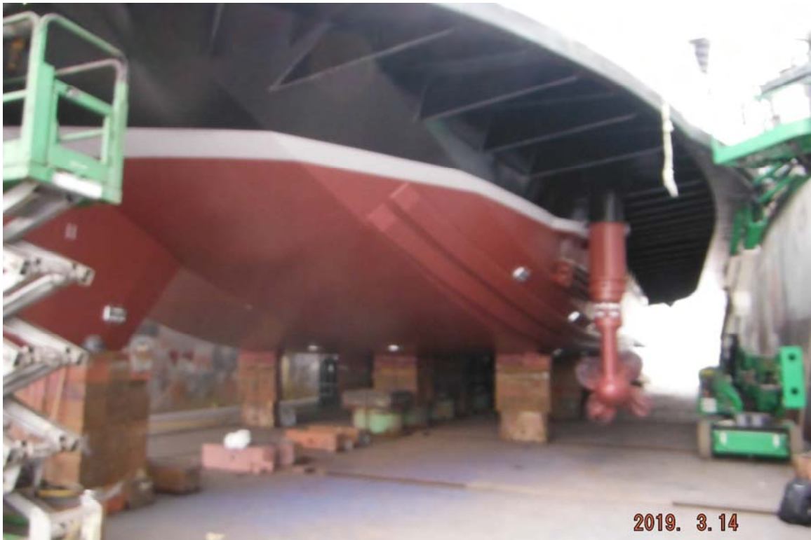
Photo No. 1 No. 1 end looking aft port side
